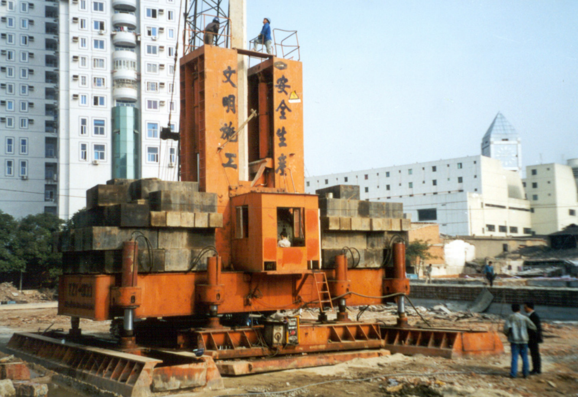
Press rig driving 550 mm concrete piles.
