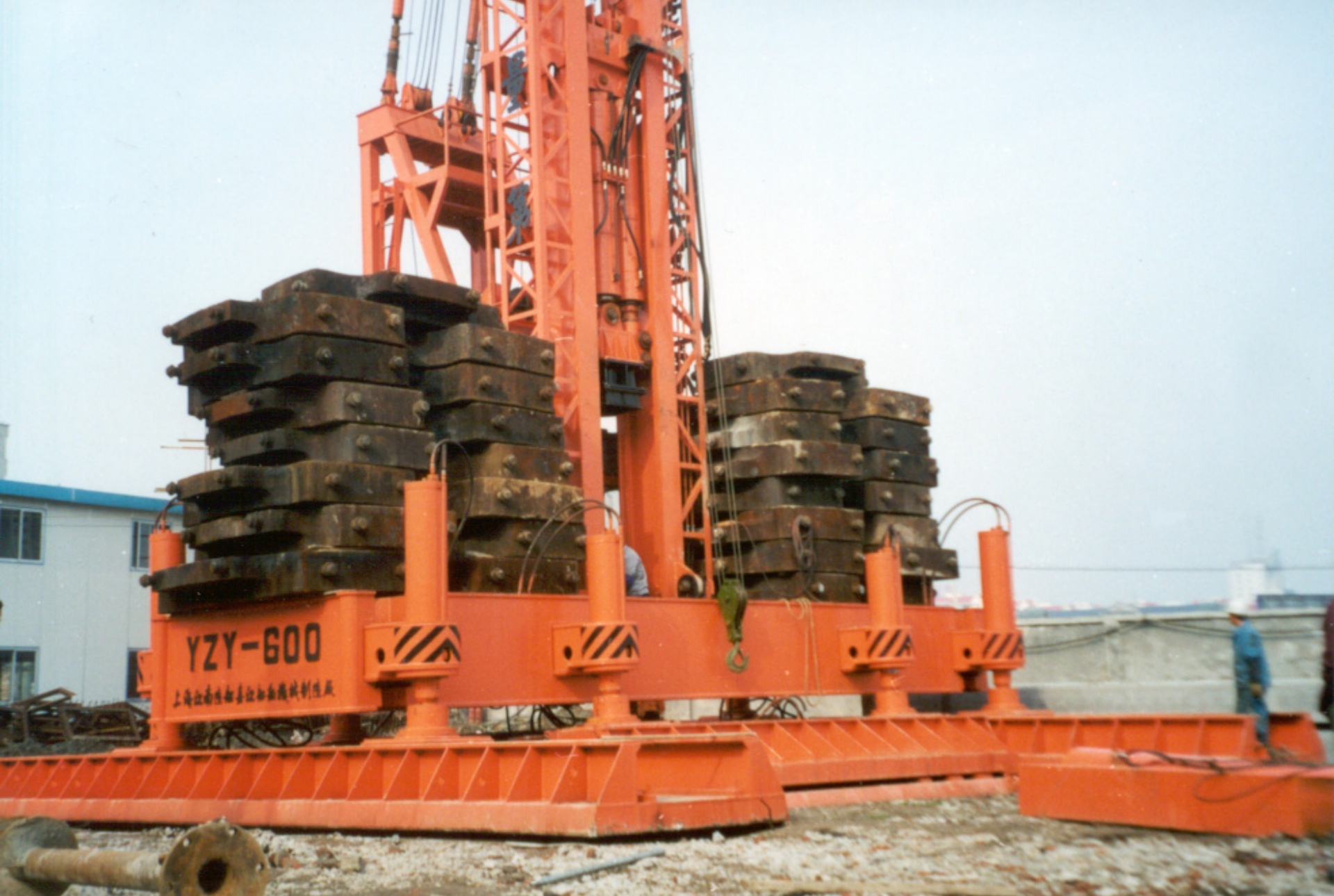
Reaction weight for 600 ton pile.
